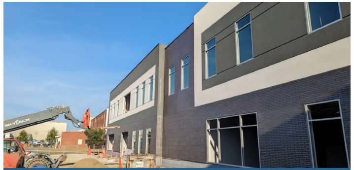
Exterior finish install working around the building
