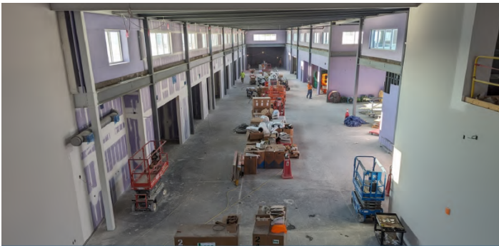
Drywall wrapping up in atrium space
