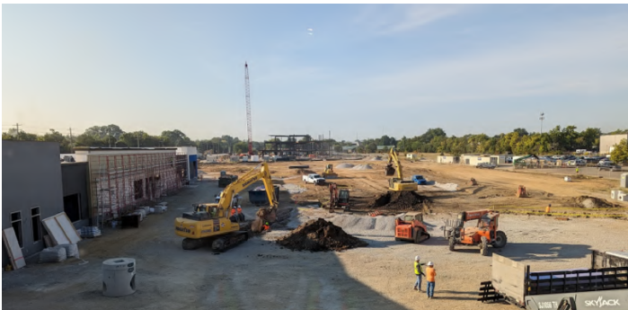
Site work has begun
